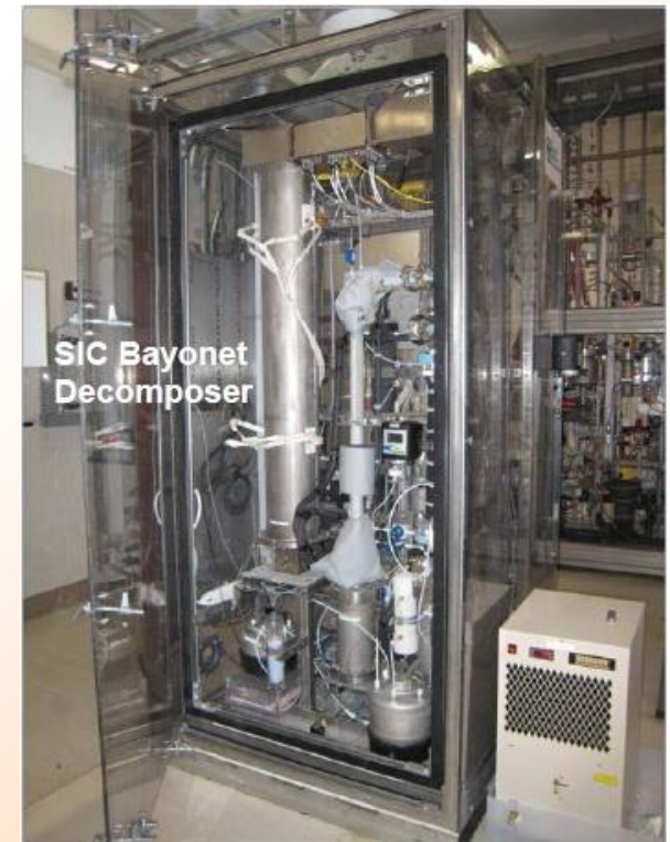
\text{H}_2\text{SO}_4 decomposer unit installed at GA ILS experiment site
